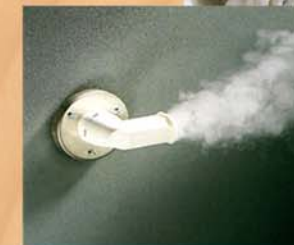
Steam room outlet emitting hot steam into the room
